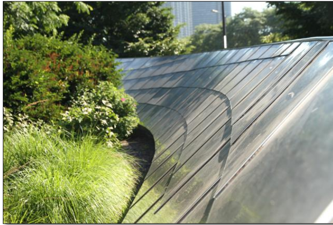
Steel plates form the exterior “skin” of the BP Bridge. Ryan Mikulenska
