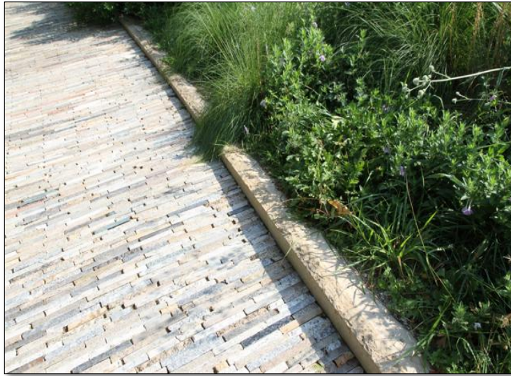
The recycled counter top walkway is one of several different paving surfaces located throughout the park. Ryan Mikulenska
