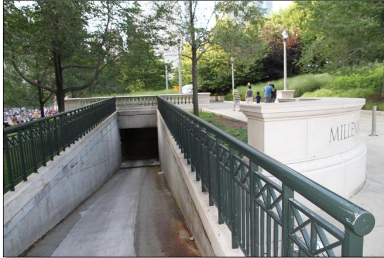
The ramp that leads to the underground trash storage facility can be seen here. Storing the trash underground helps enhance the park's smell. Ryan Mikulenska
