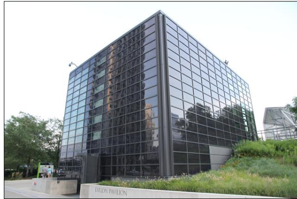
The two North Exelon Pavilions, one of which can be seen here, received a LEED Silver rating from the United States Green Building Council. Ryan Mikulenska
