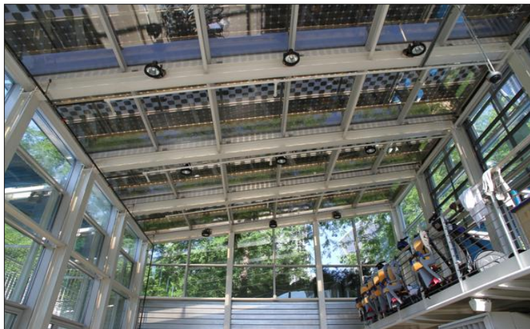
120 solar panels on the roof of the McDonald’s Cycle Center produce about 6.5% of the electricity supply required.
